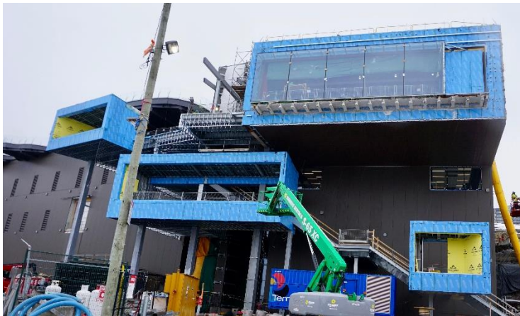
Photograph of construction at the Cliff Energy Centre, February 2024
