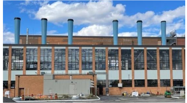
View of Confederation Heights Energy Centre showcasing the new roof and structural steel upgrades.
