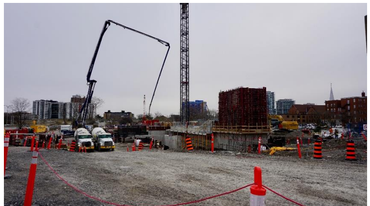
Gatineau Energy Centre's Construction 2024
