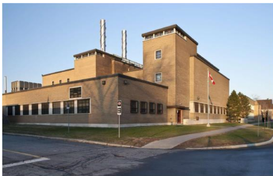
Existing Tunney's Pasture Heating and Cooling Plant, 2023
